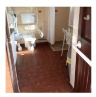
The shower area is 800mm square, with curtain around, thermostatically controlled shower with controls at 900mm height, and shower head adjustable from 750mm to 1500mm height. The shower has a drop-down seat, and fixed vertical and horizontal grab rails. The turning circle for a wheelchair user is restricted to 1100mm by the baby changing worktop.
