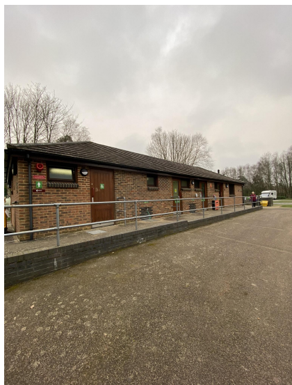
Upper Toilet Block
