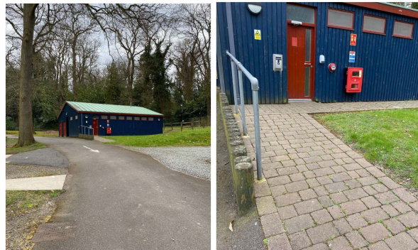
Access to Toilet Block C is via a slight slope with a handrail to one side
